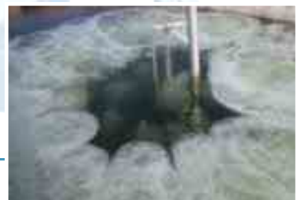
Starting stages of a radial submersible aerator.
