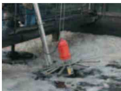
Installation stages of a submersible aerator type SCL
