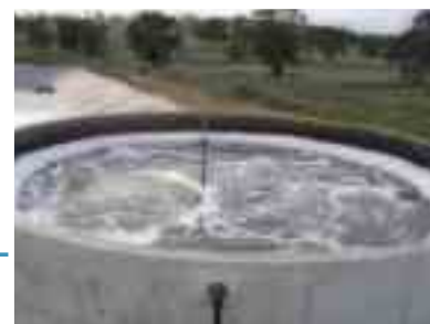
Installation of a submersible aerator type SCL
